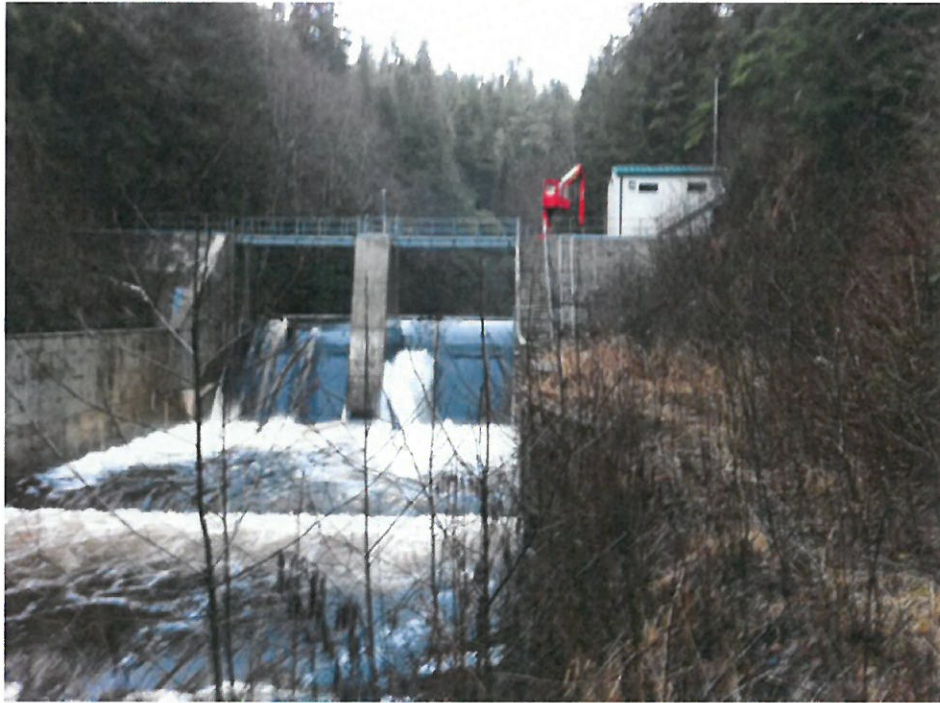
Figure 2 - Existing Dam on Gunnuk Creek
