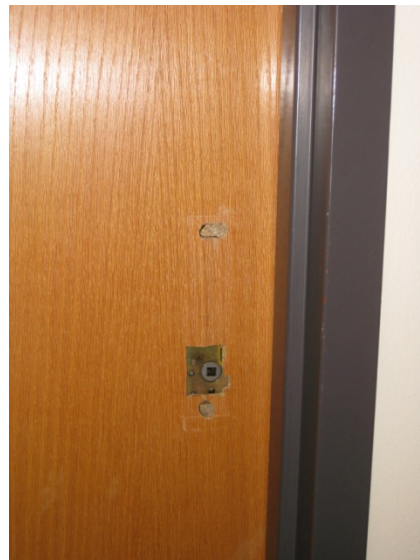
A10 Interior doors
