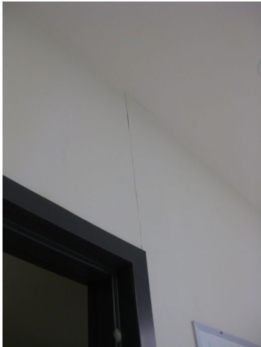
A14 OR wall covering seams
