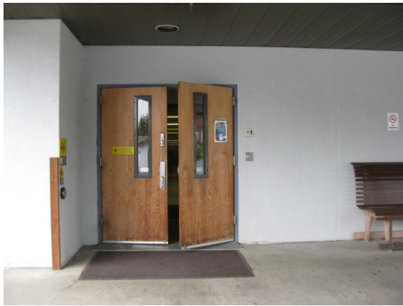
A7 Entry Door at Emergency
