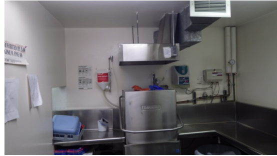
38. KITCHEN DISHWASHING ROOM
