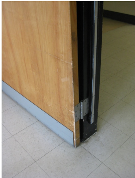
A9 Interior doors
