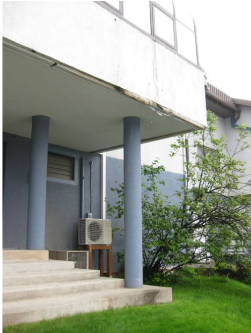
A1 Sun Room Siding
