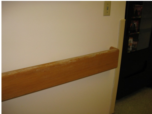
A16 Wood Railings
