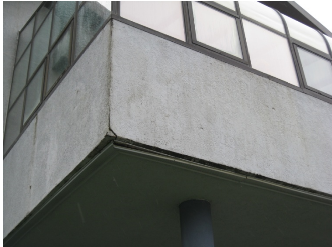
A2 Sun Room Siding
