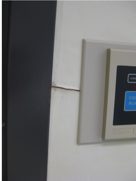
A15 OR wall covering seams
