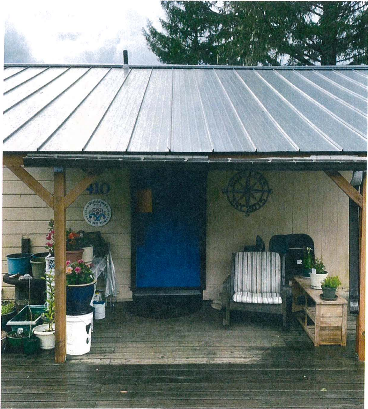
Photo of 410 Mitkof Highway showing Notice and Order of Abatement packet on front door 8/3/2020
